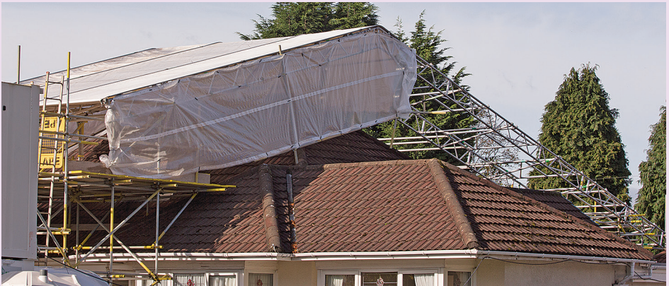
The attic conversion
